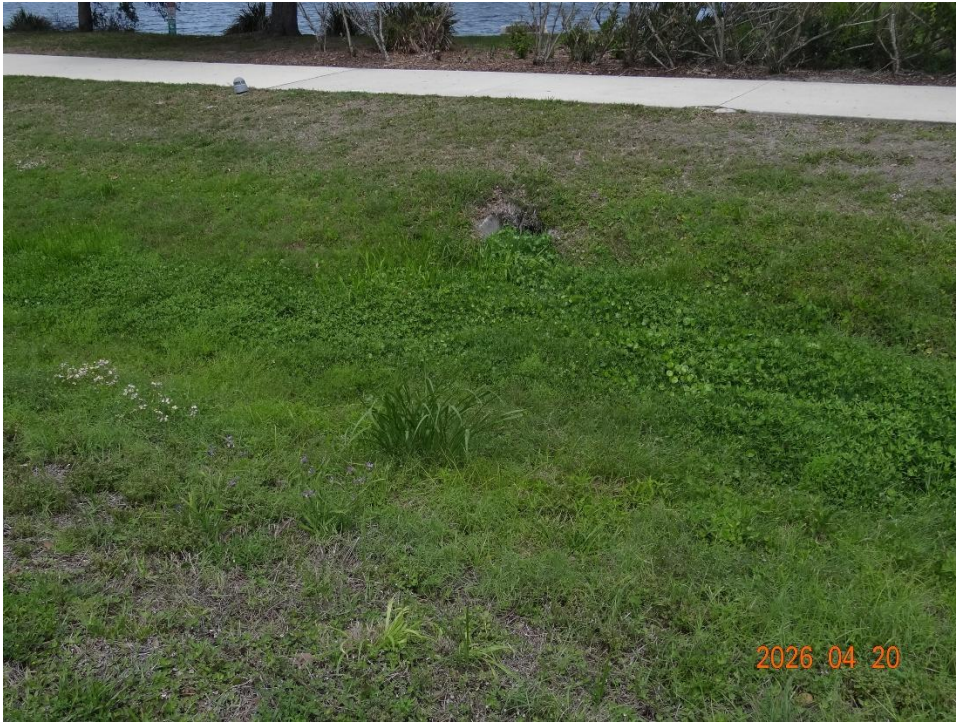
Area 1 outfall pipe from OCS 1
