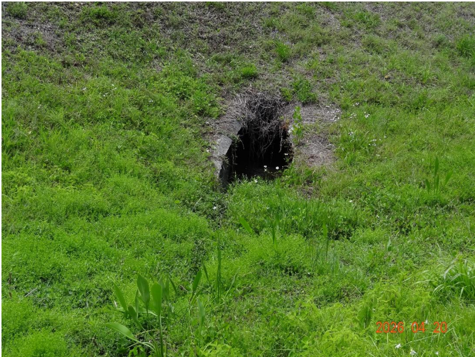
Area 1 pipe under Williamson Blvd.
