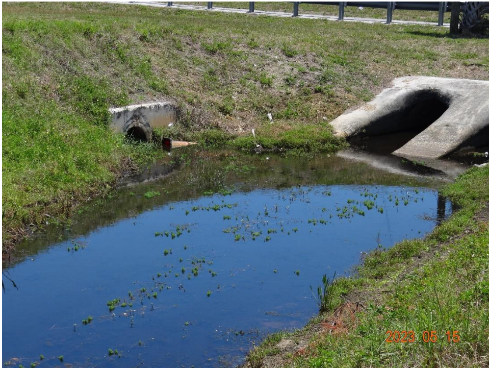
POND B OUTFALL PIPE
